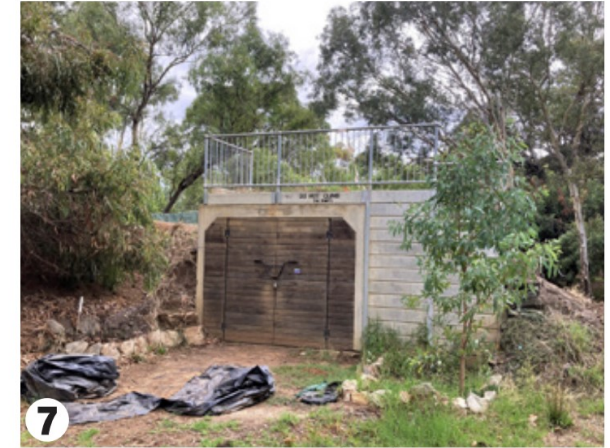
7 Culvert storage under berm with raised viewing platform over.
